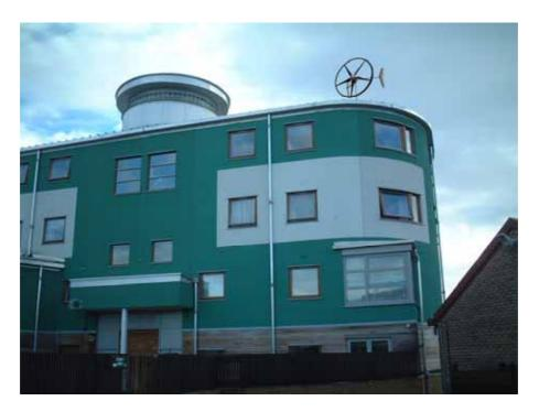
Figure 2 – A typical Swift turbine installation in a residential block
