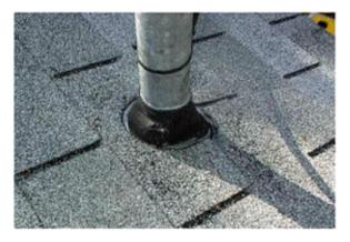
Figure 6 - Typical installation of rubber roof gland seal.
